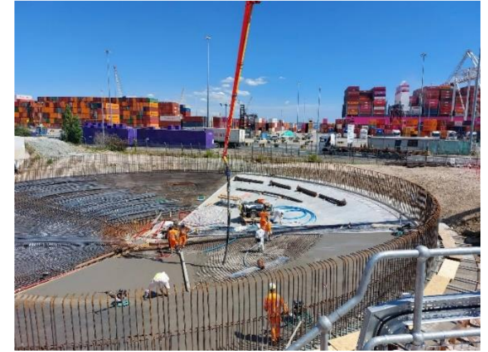
Millbrook WTW - U_IMP5 works
