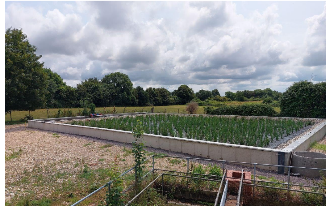
Lavant WTW wetland: using nature to prevent harm from discharges from the storm overflow
